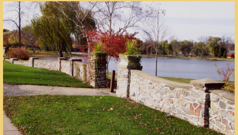
The glacial fieldstone wall at Riverside Park in Watertown, WI uses the natural, local stone
