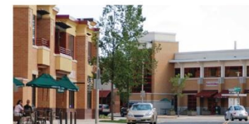
Middleton Hills, WI incorporates employment and shopping in the center with residential nearby
