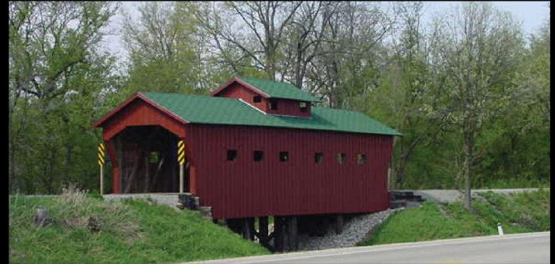
Covered bridge south of Fort Atkinson, WI, was built using boards from a nearby obsolete barn
